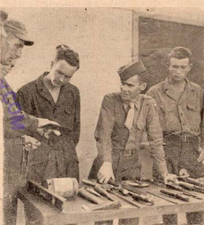
Pfc. Carl Swanson, (left) engineer utilities instructor at ECES, demonstrates the use of working tools to a class.
